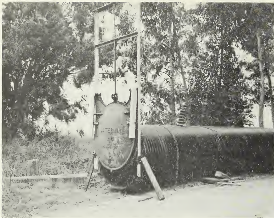
Photo 6. Asphalt coated corrugated metal pipe with attached combination slide and flap gate used as tidal water control structure.
